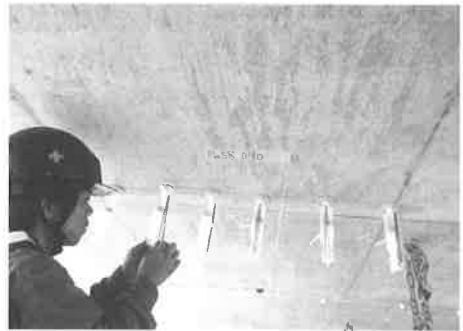
図-7 ひび割れ補修工
